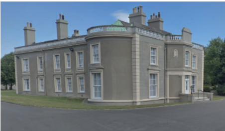
Fig. 5 - * PROTECTED STRUCTURE SYBIL HILL HOUSE/ VINCINTIAN PROVINCIAL HOUSE
