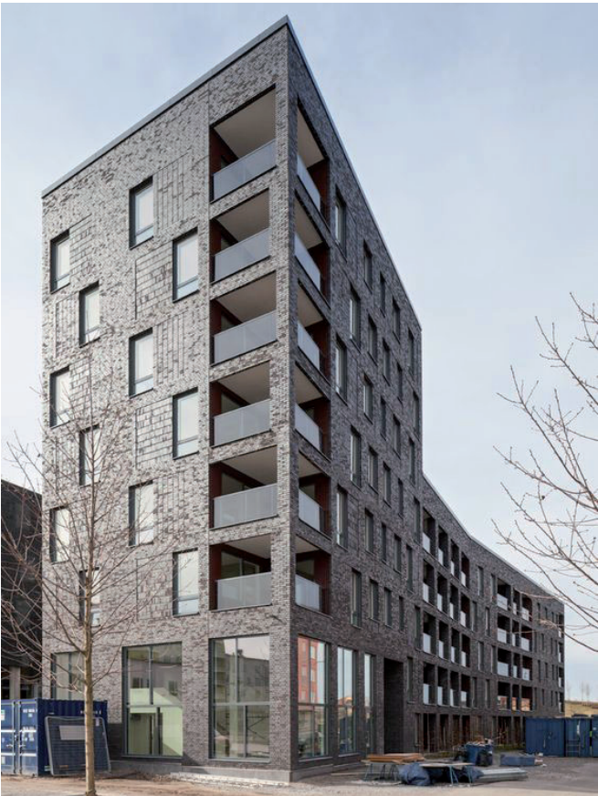
Fig. 63 - Long block steps down from 7 Storey to 5 storey providing relief and drawing the eye along its length for horizontal emphasis
