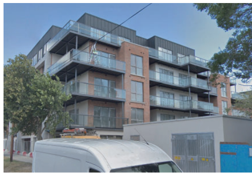
Fig. 4 - ARDILAUN COURT RESIDENTIAL DEVELOPMENT. CURRENTLY UNDER CONSTRUCTION WITH 76 NO. APARTMENTS AND HOUSES. CURRENTLY UP TO 5 STOREY APARTMENT BLOCKS WITH PLANNING APPROVAL FOR 6TH FLOOR.
