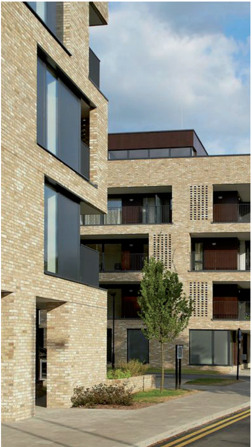
Fig. 64 - Wrap around windows and balconies
